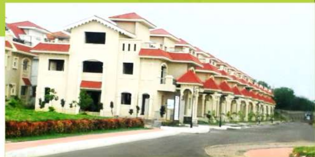
STREET VIEW PHOTO SHOT AT SITE
